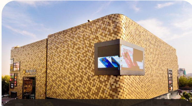
Palladium Mall, Ahmedabad
