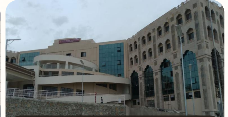
Hospital Project In Udaipur Rajasthan
