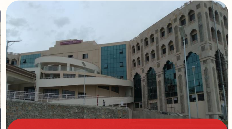
Hospital Project In Udaipur Rajasthan
