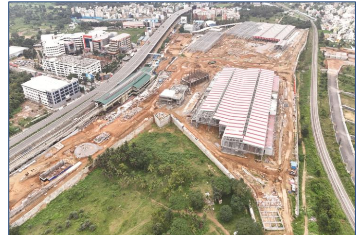
Challaghatta metro depot cum workshop, Karnataka
