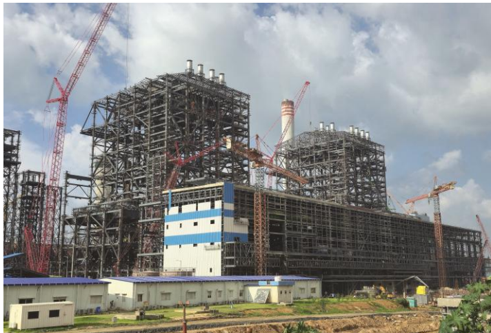
2 X 800 MW Mahan Ultra SCTPP, Madhya Pradesh
