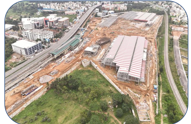
Challaghatta metro depot cum workshop, Karnataka
