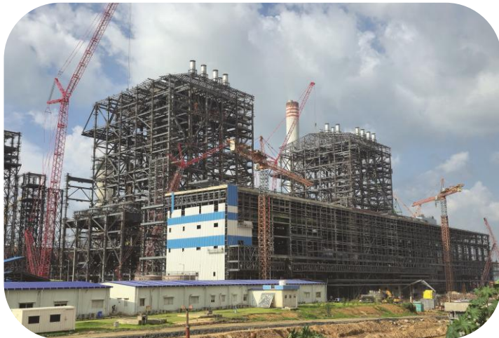
2 X 800 MW Mahan Ultra SCTPP, Madhya Pradesh
