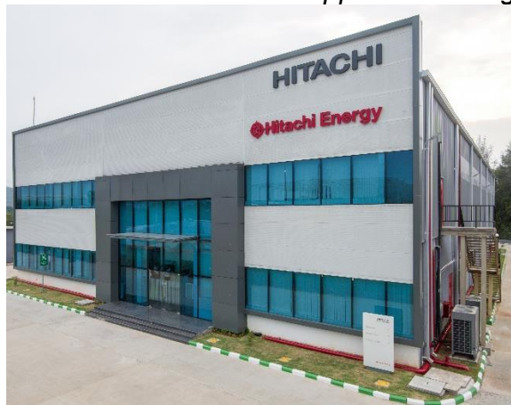
The HVDC and Power Quality factory in Chennai
