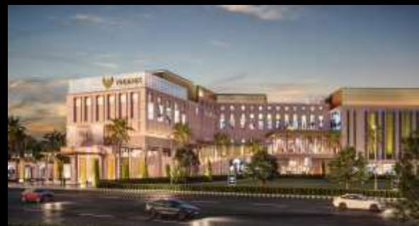
Under-development mall at Kolkata
