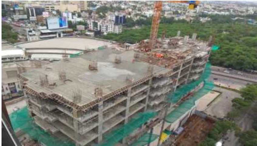
Fountainhead Tower 2 - Side
