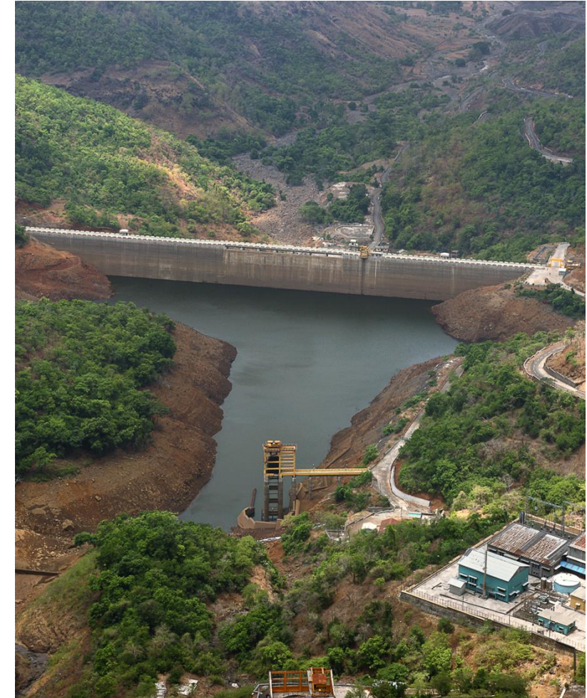
Ghatghar Dam - Maharashtra 84m high 10th fastest completed dam in the world & India's first RCC Dam
