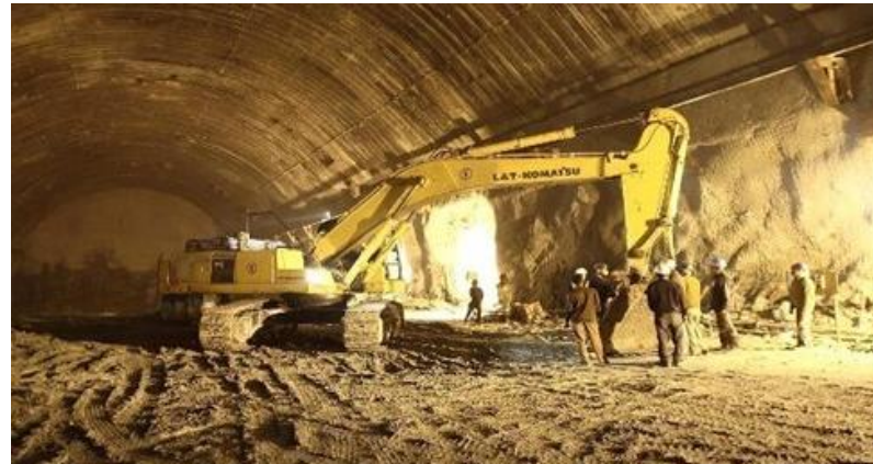
Srisaillam HE Project - Andhra Pradesh (900 MW) Largest Underground Cavern in Asia 25.7m (W) x 53m (H) x 236m (L)
