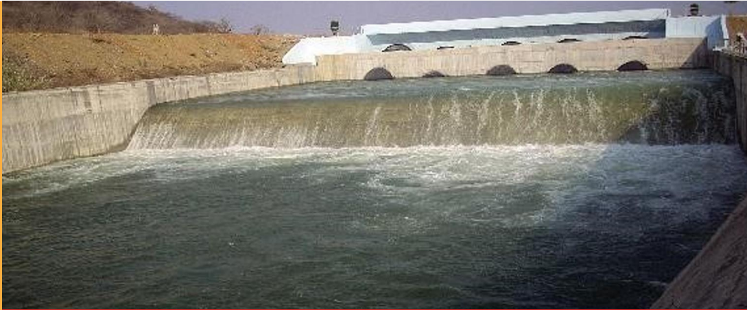
Kalwakurty Lift Irrigation Project, Andhra Pradesh
