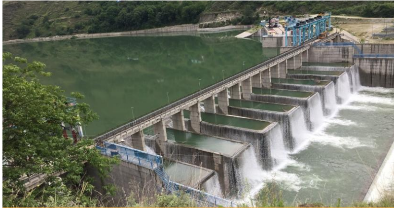
Sawrakuddu HE Project - Himachal Pradesh (111 MW) First Piano Key Weir in India
