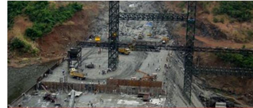
Roller Compacted Concrete (RCC)
