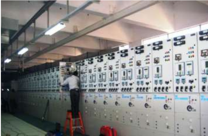
33KV AIS Replaced with 33KV GIS at Essar Oil, Jamnagar Refinery (2011)
