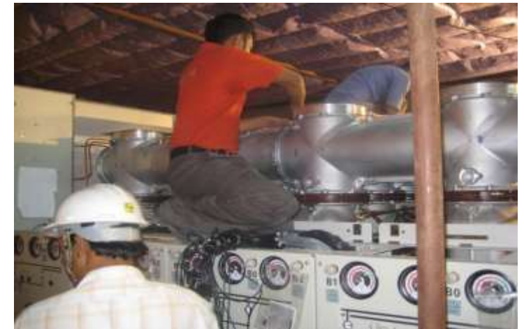
Precision Installation of GIS at IOCL-Panipat Refinery (2008 – 2009)
