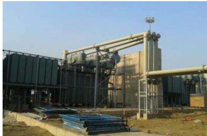
220KV GIS Installation with GIB Connection to Transformers at Tata Steel, Kalinga Nagar, Odisha
