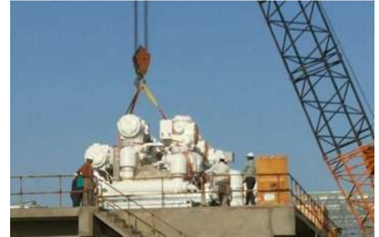
220KV GIS Installation on Terrace at 250MW Power plant in Mundra, Gujarat
