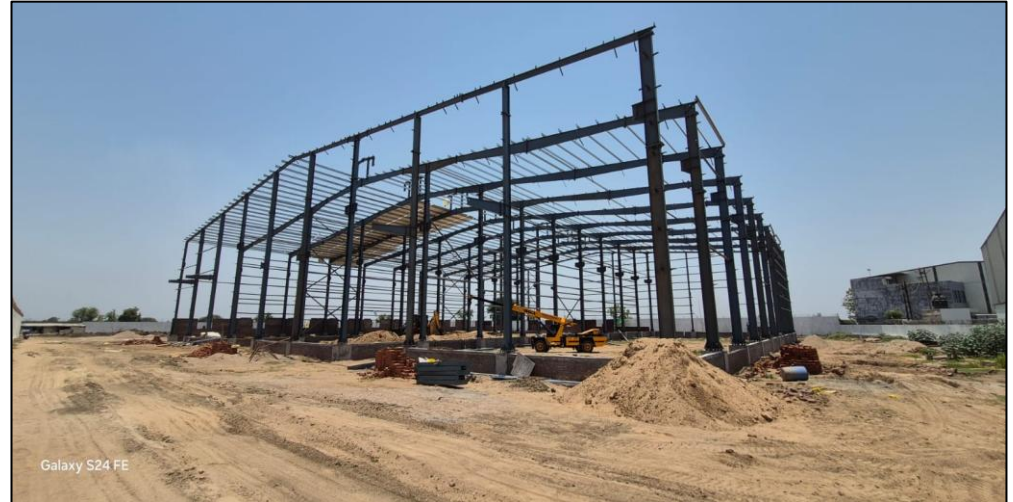
Front View of Manufacturing Shed
