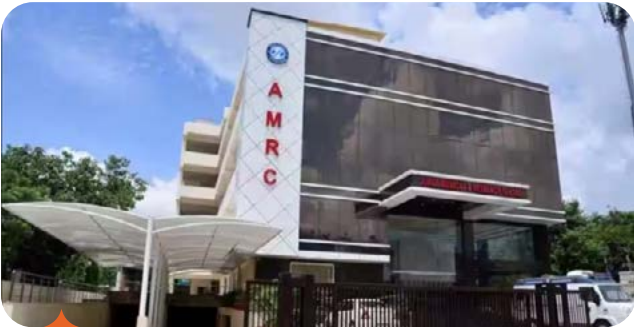
Amar Medical & Research Centre Jaipur Before ● ₹ 5 Mn / month (Feb-2022) At the time of acquisition
