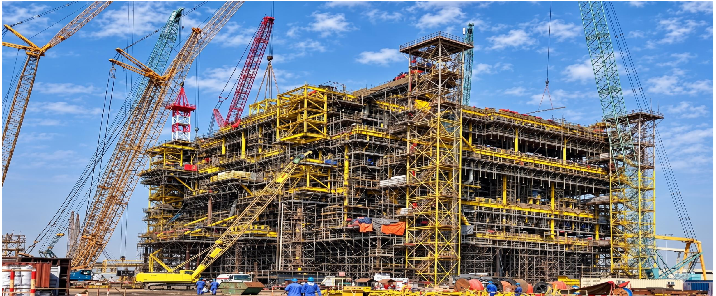
Fabrication at Sohar Yard (Oman) of Riser Platform for North Oil Company's Ruya Development (Qatar) Project
