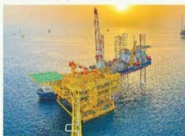
Setting Global Benchmarks: Hasbah-II Offshore Project, KSA
