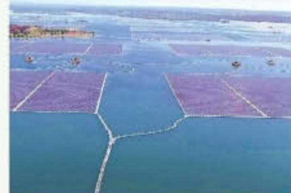
India's Largest Floating Solar Project, Madhya Pradesh
