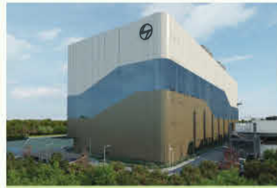
Data Center in Sriperumbudur, Tamil Nadu
