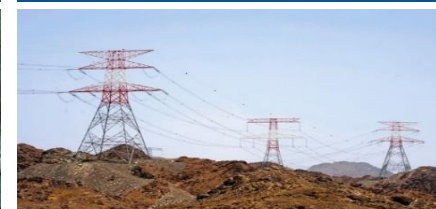
Transmission Lines, Fujirah, Dhaid
