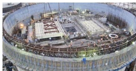
Kakrapar Nuclear Power Plant, Guj
