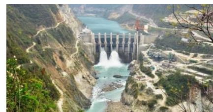
Srinagar Hydro Electric Plant
