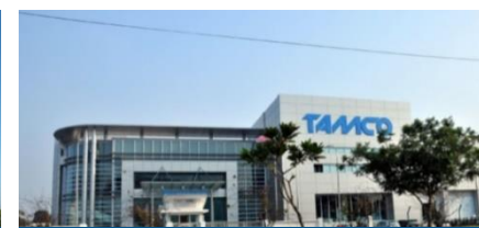
MV Switchgear Factory, Malaysia
