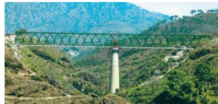
88m Rail Bridge Jammu Udhampur
