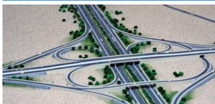
Sheikh Khalifa Interchange, UAE
