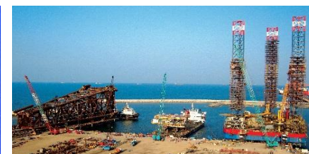
Fabrication Facility, Oman
