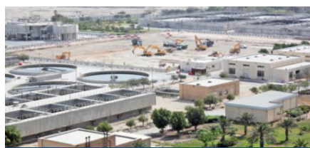
Water Treatment Plant, Doha
