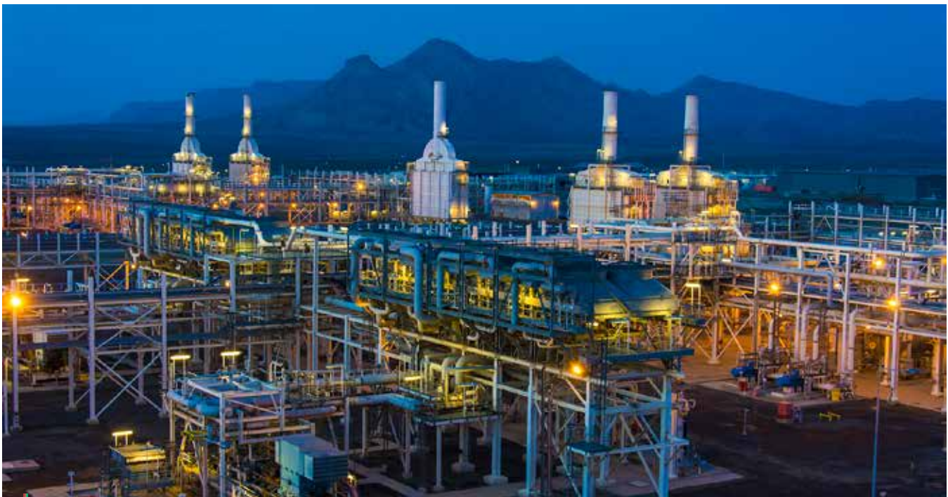
Sangachal: Powering progress across borders
