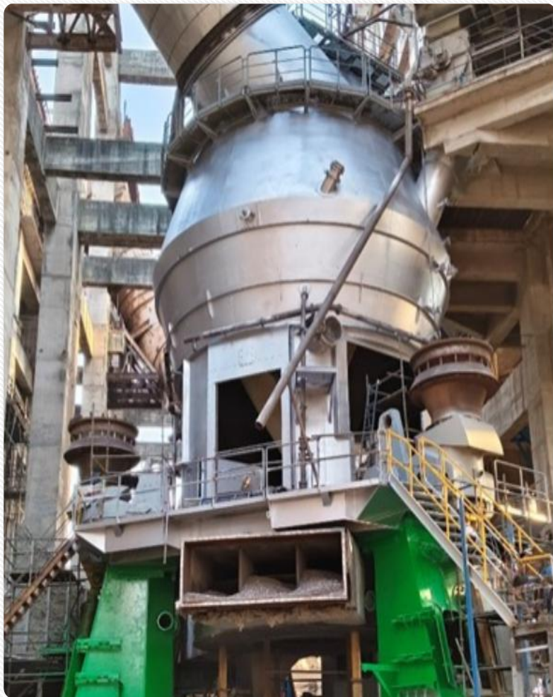
Cement VRM upgradation on track
