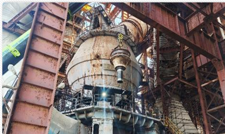
Raw Mill modernization work-in-progress
