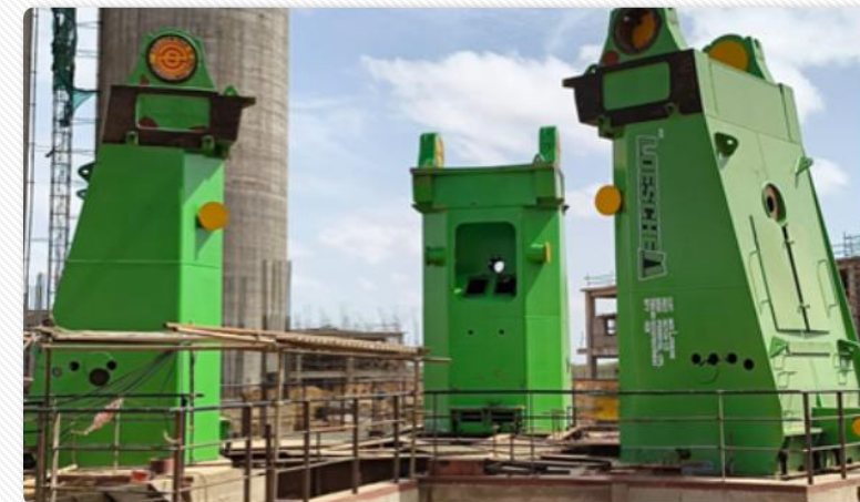
VRM installation commenced
