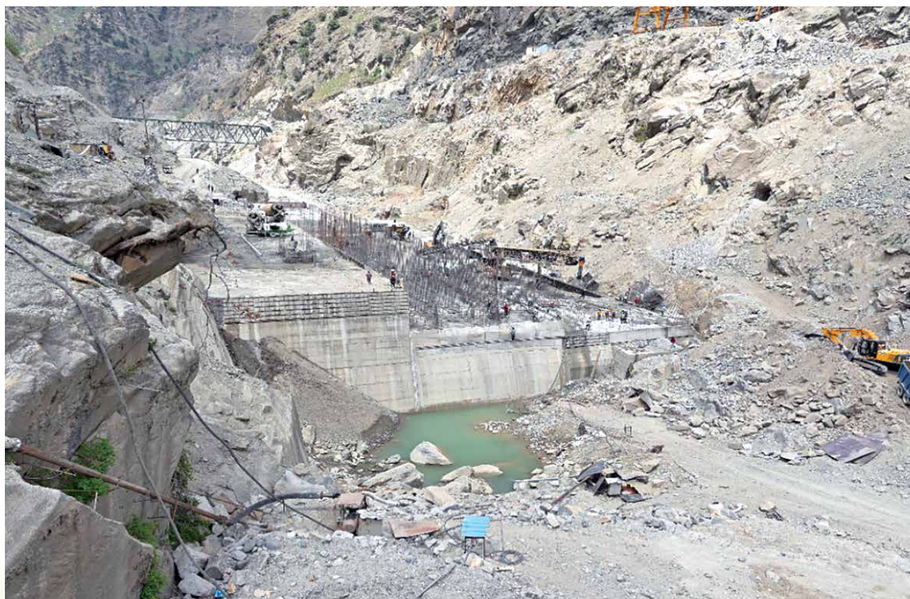
DAM CONCRETING – 540 MW KWAR PROJECT (UT OF J&K)
