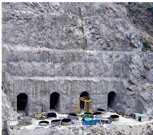
POWER INTAKE – 850 MW RATLE PROJECT (UT OF J&K)
