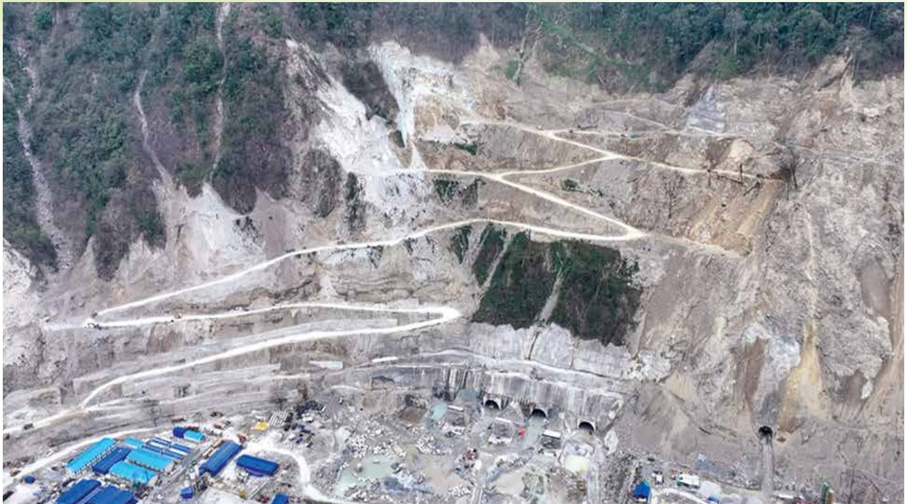
DIVERSION TUNNEL OUTLET 1 TO 5 - 2880 MW DIBANG MULTIPURPOSE PROJECT (ARUNACHAL PRADESH)
