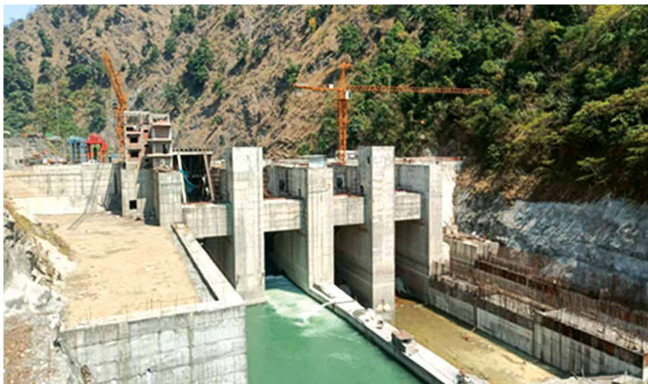
DOWNSTREAM VIEW OF DAM – 120 MW RANGIT-IV PROJECT (SIKKIM)
