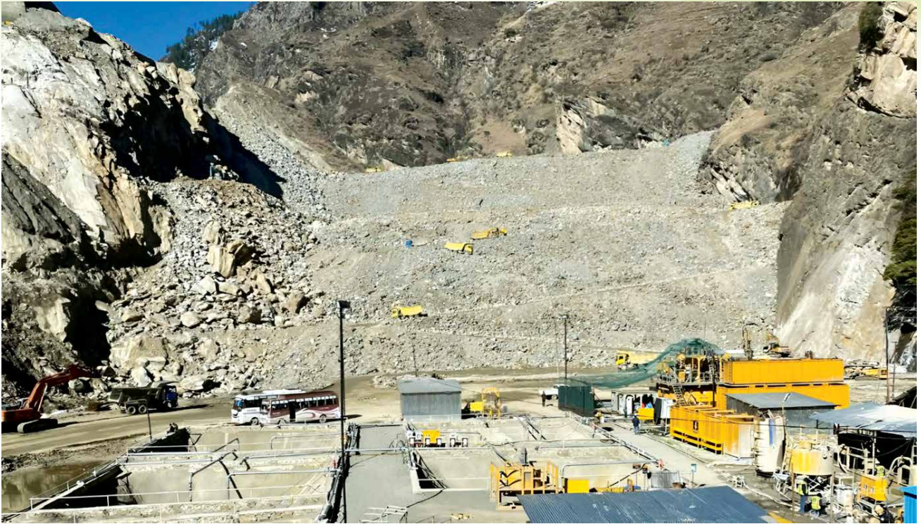
CFRD DAM FILLING – 1000 MW PAKALDUL PROJECT (UT OF J&K)
