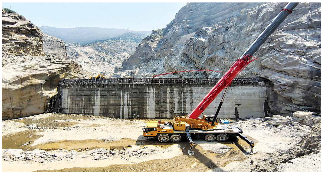
CONSTRUCTION OF COFFER DAM – 850 MW RATLE PROJECT (UT OF J&K)
