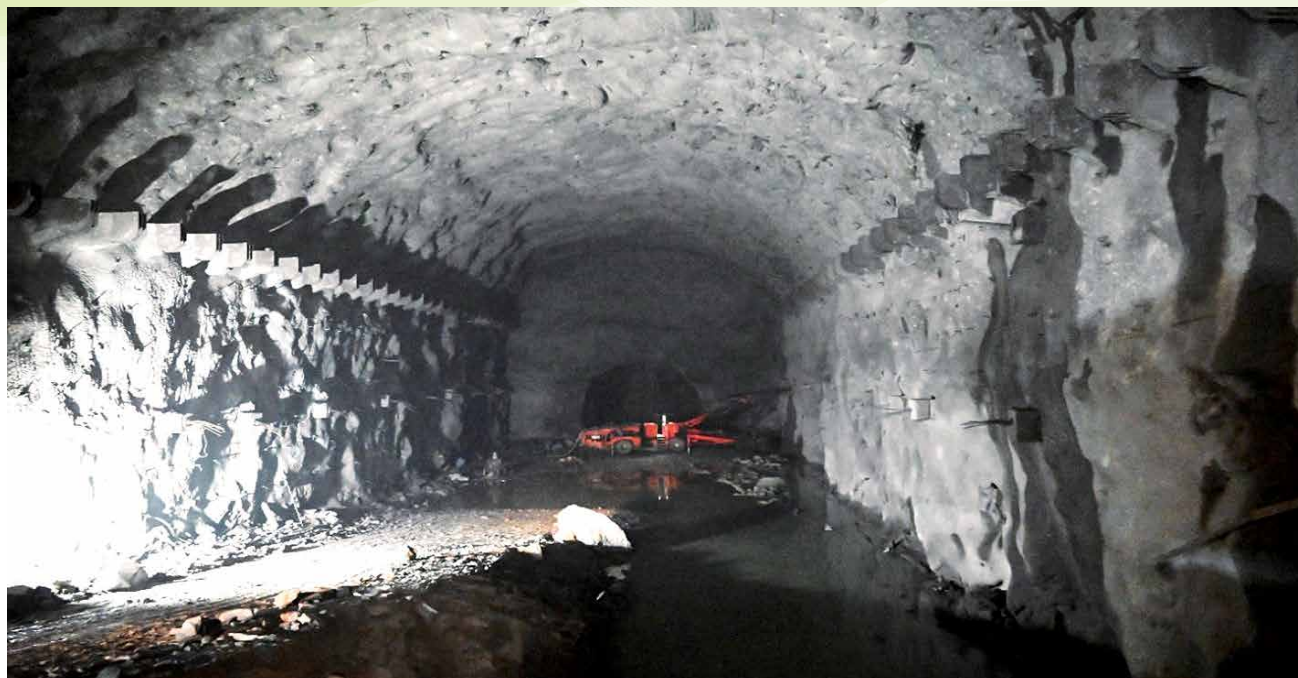
POWER HOUSE EXCAVATION – 540 MW KWAR PROJECT (UT OF J&amp;K)
