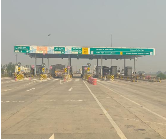
Odhaki Paipkhar Toll Plaza
