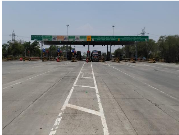
Boharipar Toll Plaza
