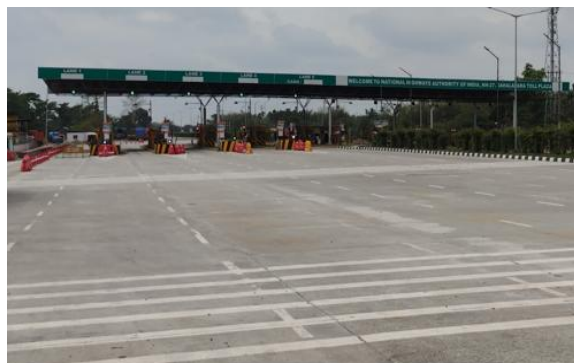
Dahalapara Toll Plaza
