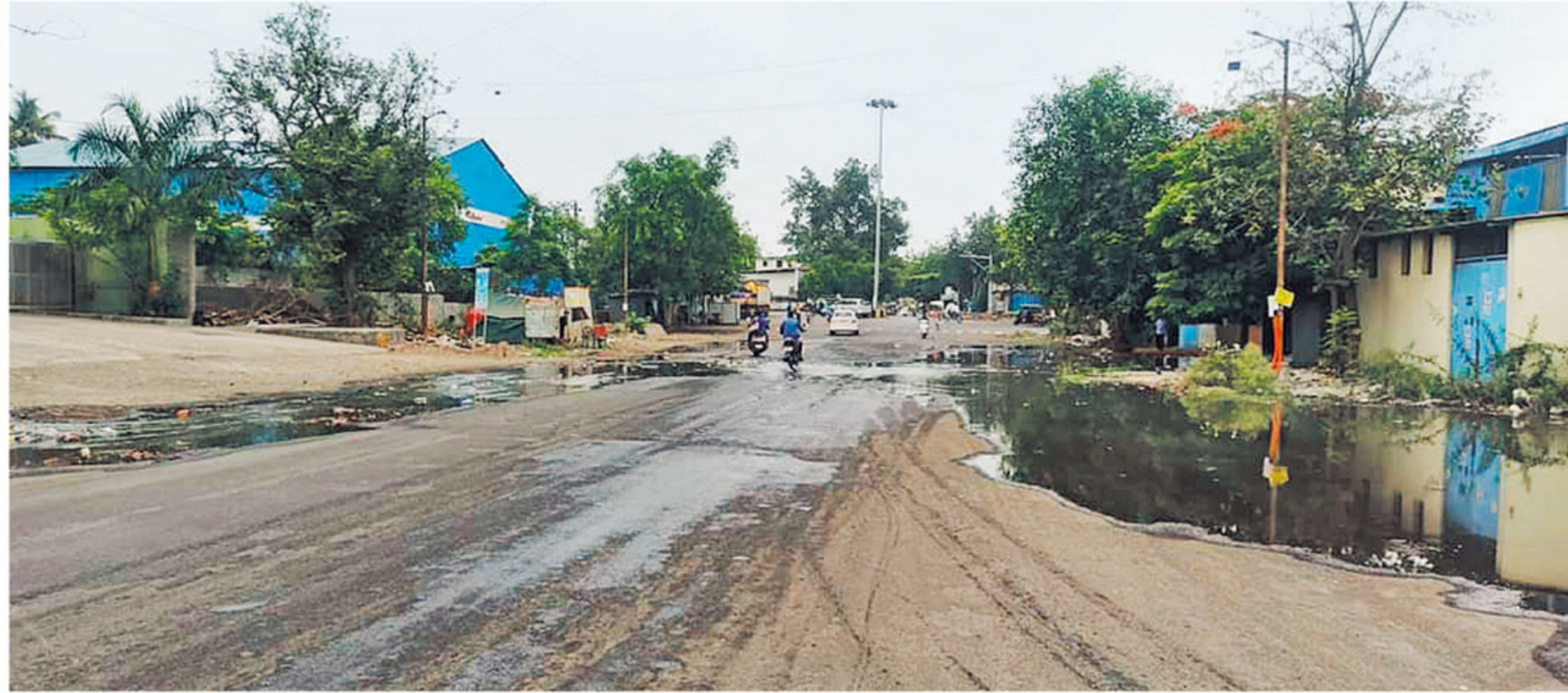
After years of wait and repeated requests, a dedicated fire station for Bhosari industrial zones is set to come up. PIC/BY SPECIAL ARRANGEMENT
