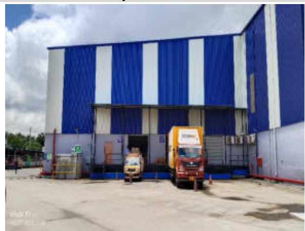
84) View of Loading Point
