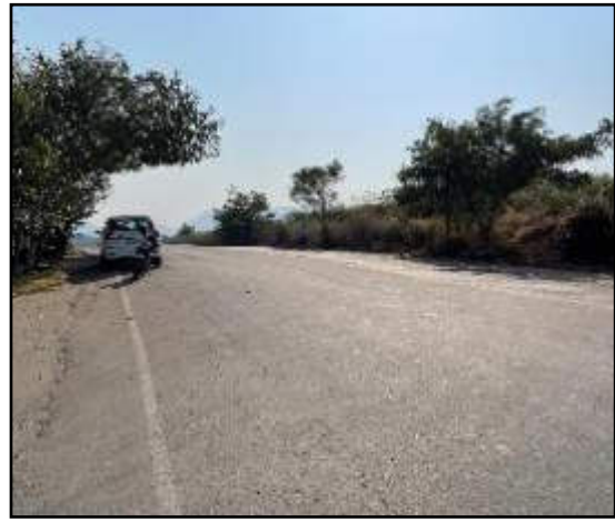
137) Access Road towards Chirner
