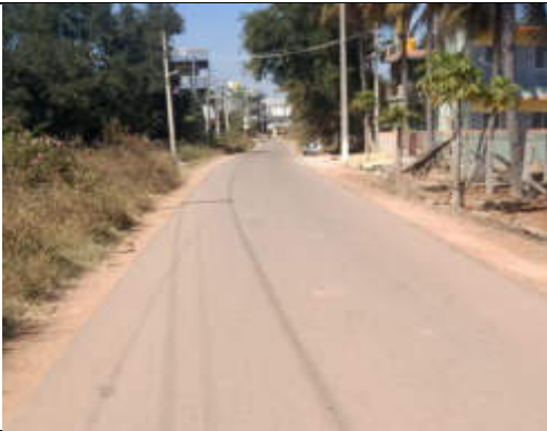
52) Access Road towards Village
