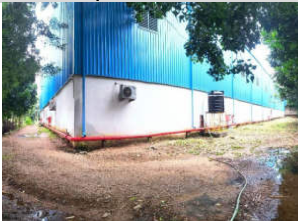
43) External View of Block
