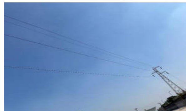
9) View of high-tension line crossing at site
