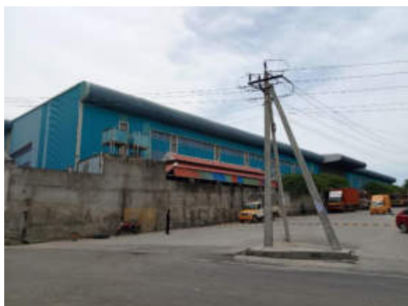
11) View of Subject Asset Compound Wall
