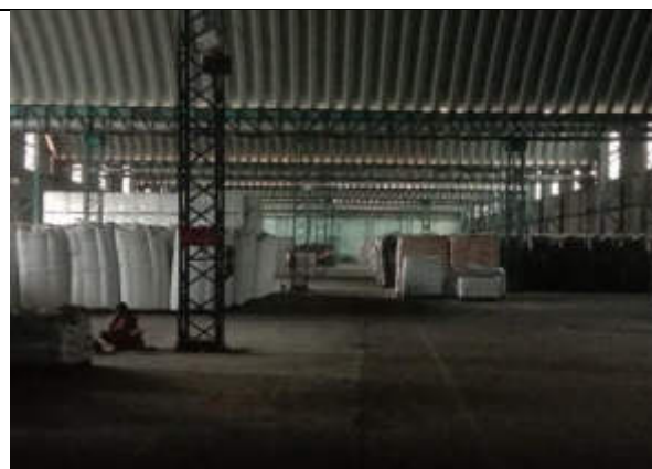
8A) View of Subject Asset
