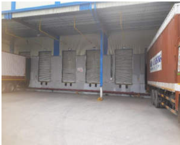
24) Dock Yard – Loading Point
