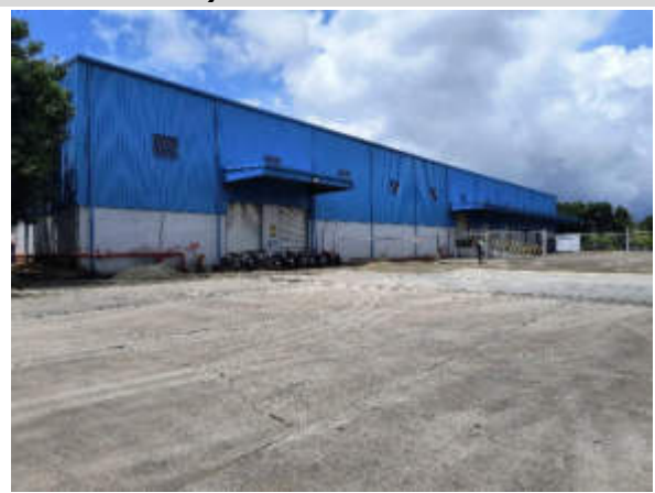
44) External View of Block
