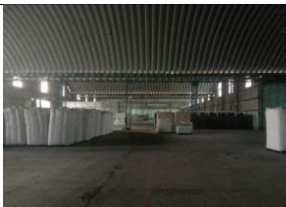
7) 7A) View of Subject Asset
