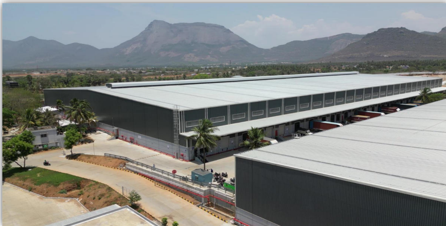
NDR Space, Thirumalayampalayam (Coimbatore) | 0.57 msf
