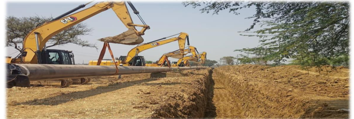
Setting up slurry pipeline
