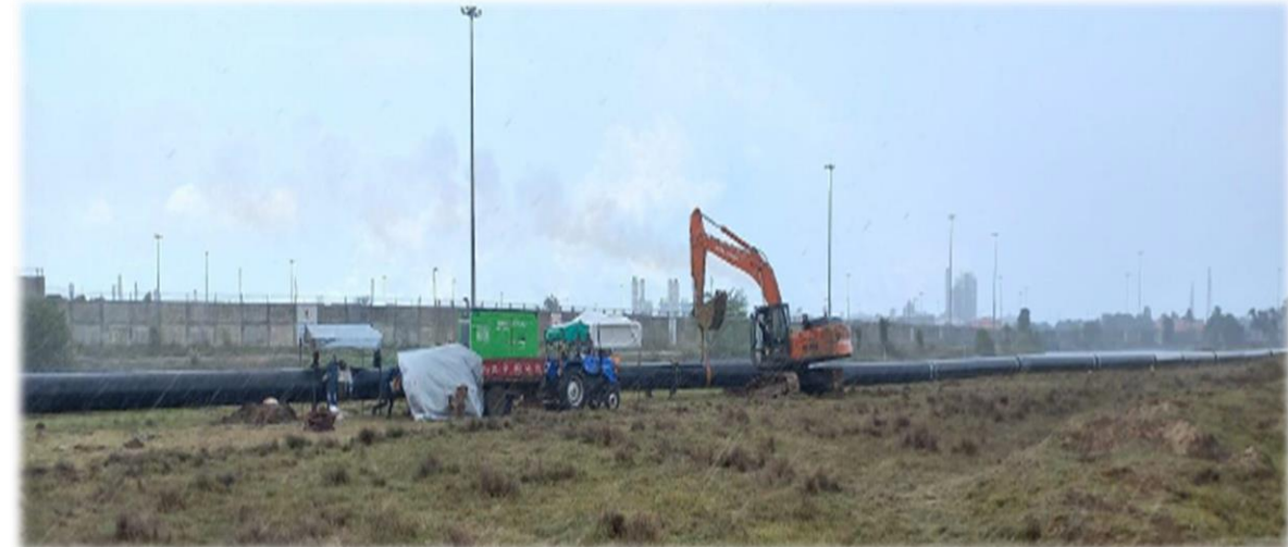
Setting up slurry pipeline
