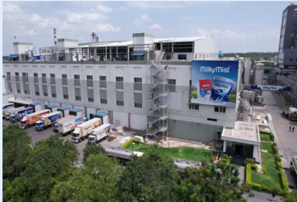
PERUNDURAI, ERODE FACILITY
