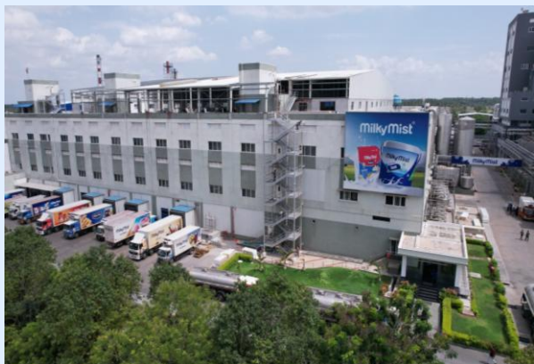
PERUNDURAI, ERODE FACILITY
