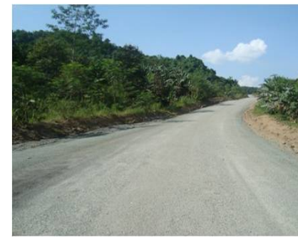
All weather haul road
