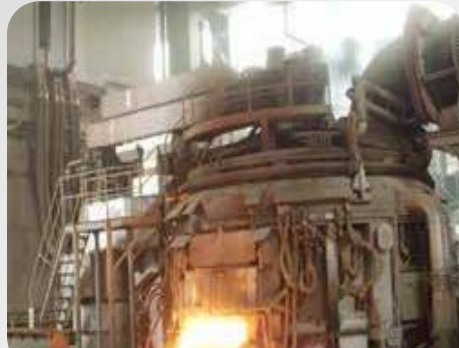
Electric Arc Furnace
