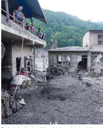
People stand amid mud and debris outside damaged structures in the aftermath of devastating flash floods in Dhangadhi district, Nepal
