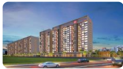
Kohinoor Projects, Pune
