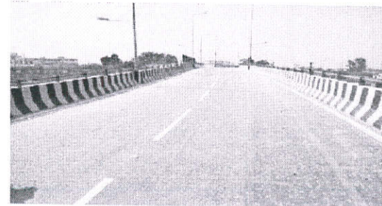
Construction of 2 lanes at Sonapat
