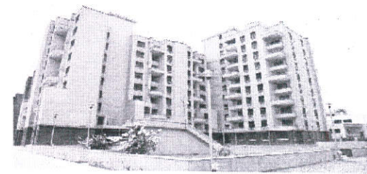
Construction of 222 Flats at Keelandev tower, Bhopal
