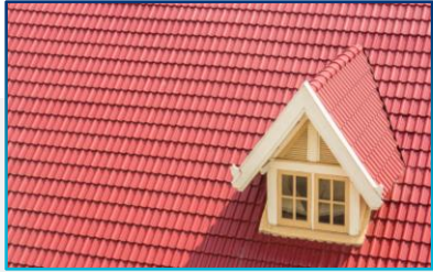
Domestic Roofing & Cladding
