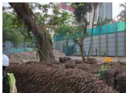
Green cloth covering, site barricading
