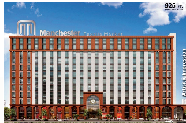
Manchester Textile Market, a large modern building with a glass facade, set to become a future-ready commercial hub.
