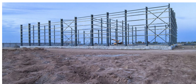
Structural steel frame at Sanosara, April 2026.
