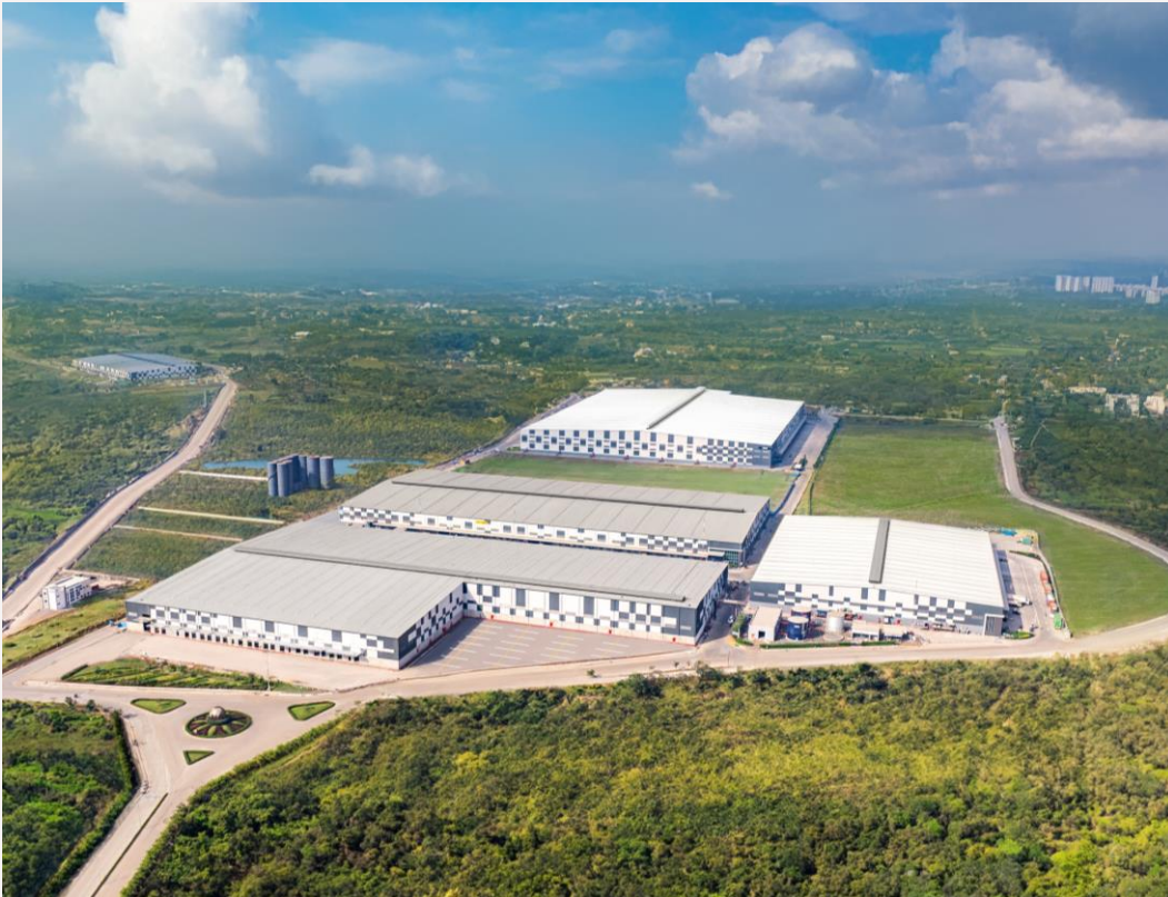
One of MMR's largest warehousing parks - Palava
