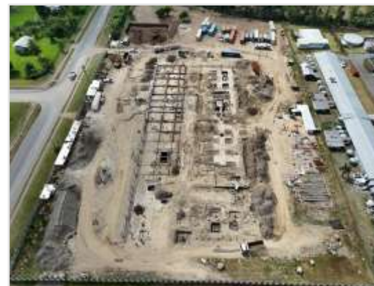
Hospital Construction Progress
