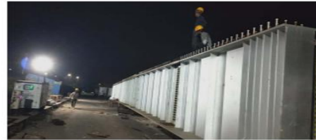
Paldi Station Metro Rail Project, Gujarat
