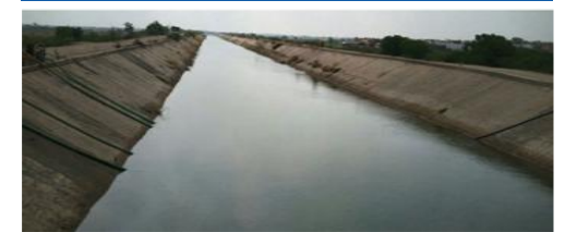
Dhrangadhra Branch Canal Work, Gujarat
