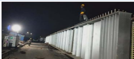
Paldi Station Metro Rail Project, Gujarat
