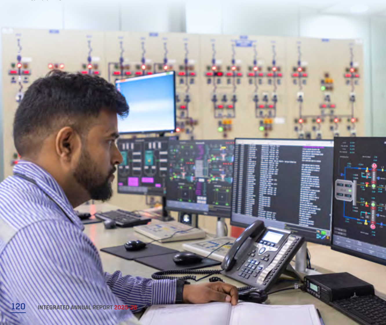
JSW Energy Vijayanagar Power Plant
