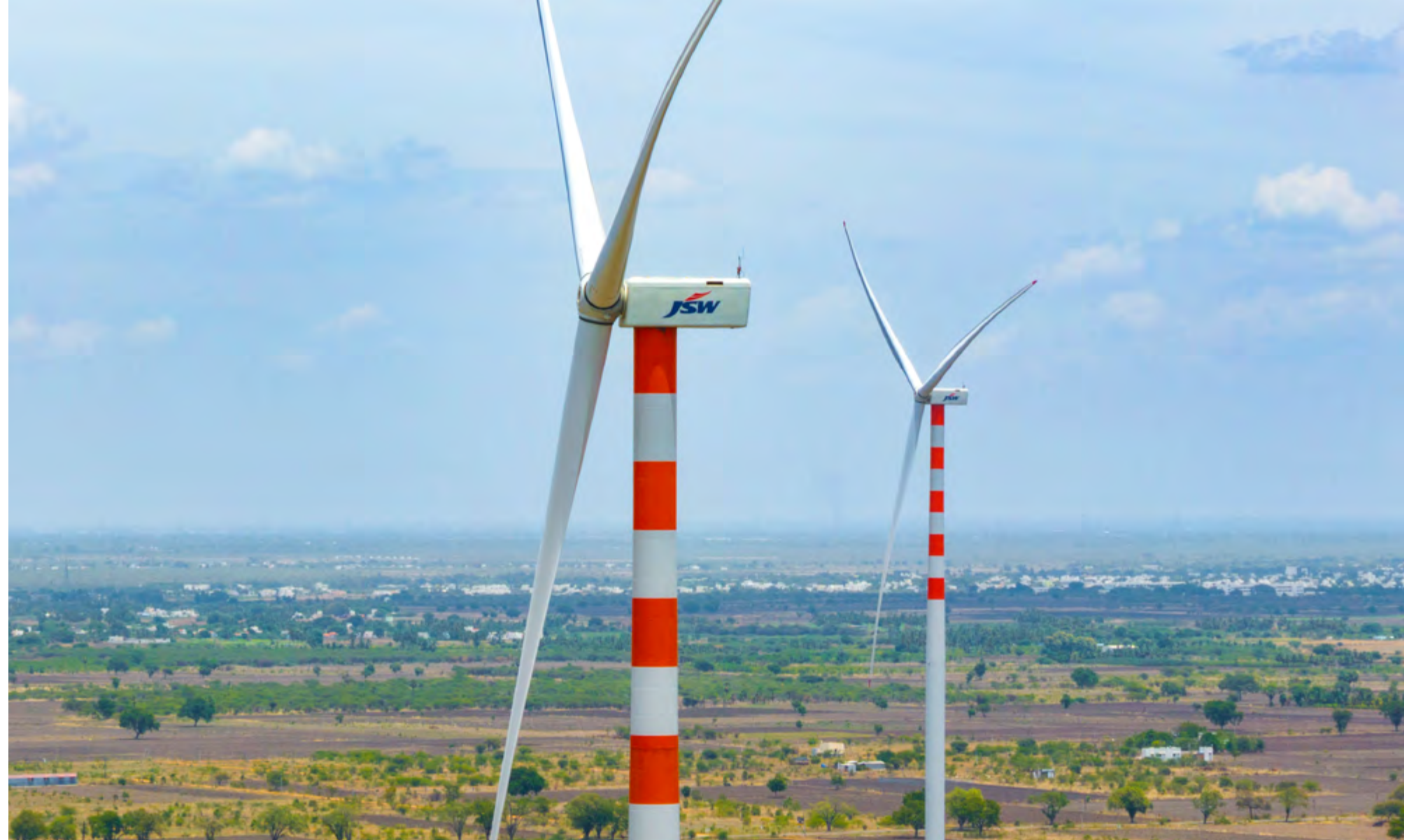
JSW Wind Energy Tuticorin Power Plant
