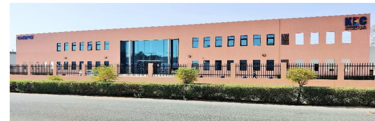
Tower Manufacturing - Dubai
