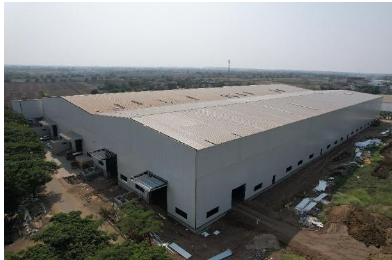
New Assembly Lines
