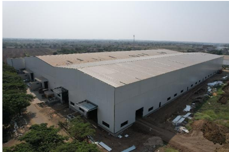
New Assembly Lines
