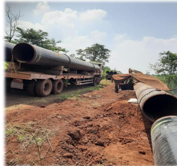
Works under progress for setting up slurry pipeline
