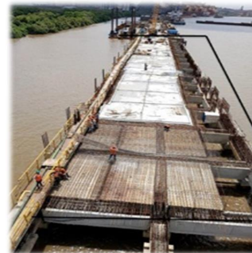
Expansion work at Dharamtar Port
