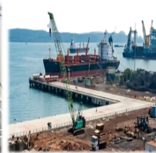
Expansion work at Jaigarh Port
