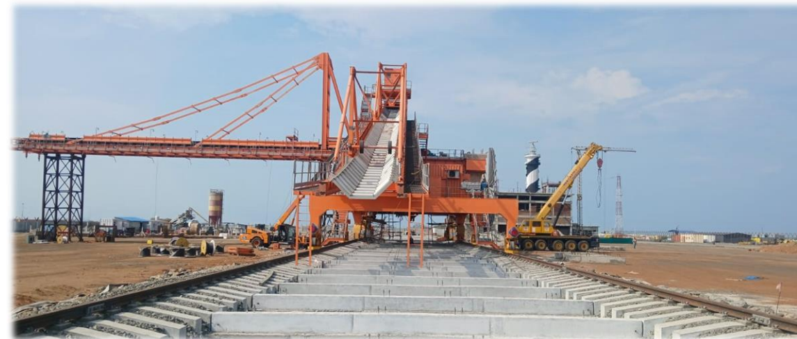
Stacker foundation and Machine erection work under progress at Tuticorin site
