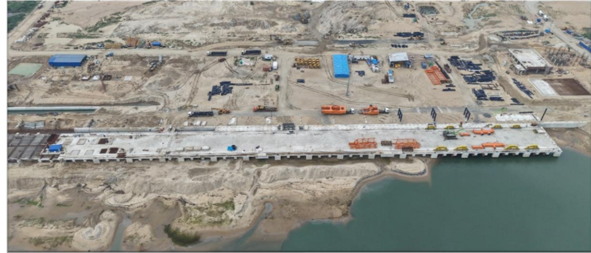
Works under progress at Jatadhar site
