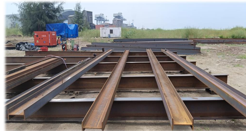
Steel fabrication for pipe rack structure at Jaigarh site
