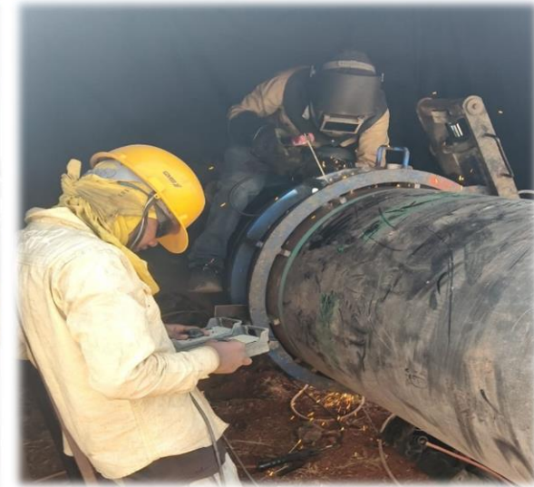
Works under progress for setting up slurry pipeline
