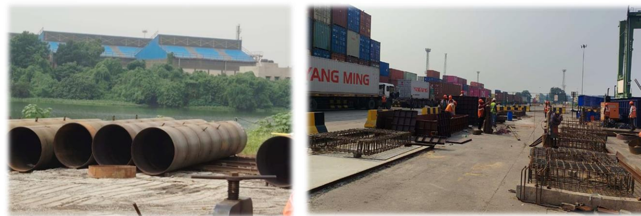
Work in progress at Kolkata site
