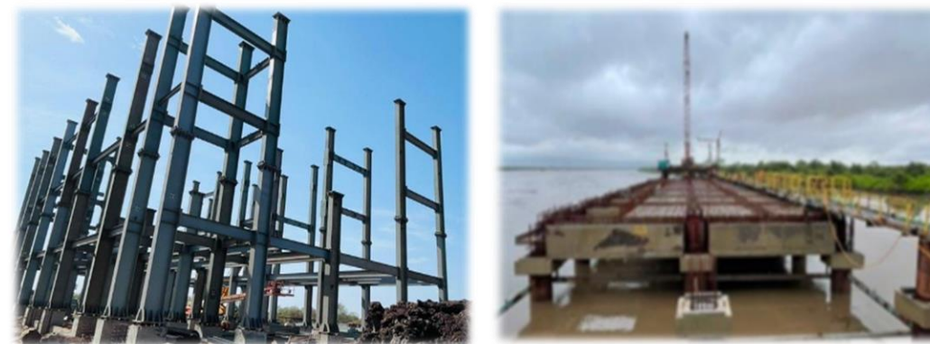
Expansion work at Dharamtar Port
