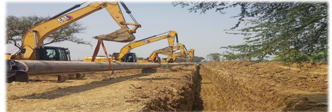
Setting up slurry pipeline
