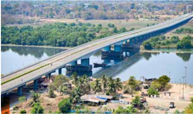
Motagaon Creek Bridge
