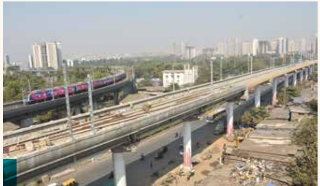
Mumbai Metro Line 9
