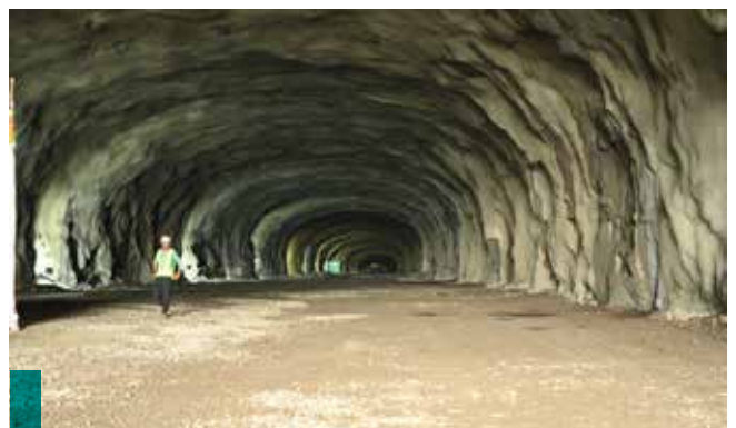
Vadodara Mumbai Expressway, IRCON
