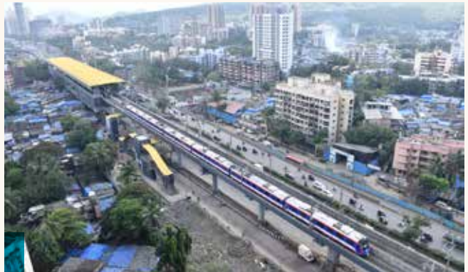
Mumbai Metro Line 7
