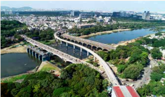
Pune Elevated Metro
