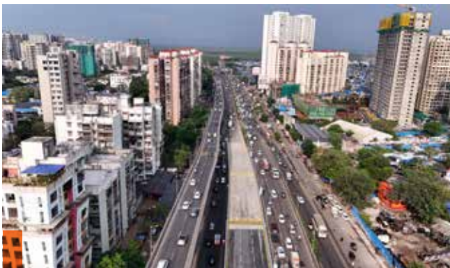
Chheda Nagar Flyover Part 1
