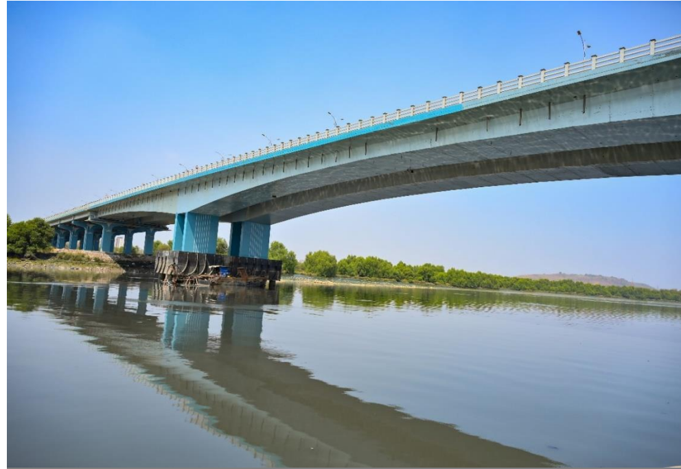
Motagaon Creek Bridge
