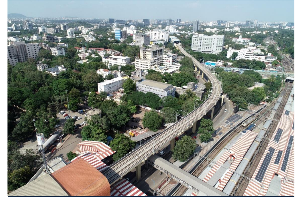
Pune Elevated Metro
