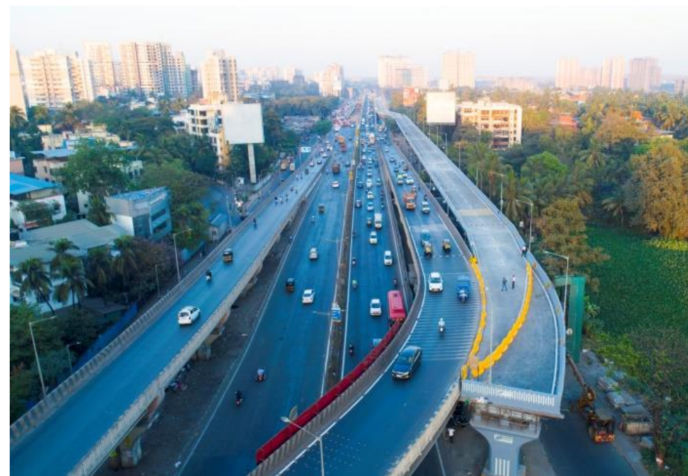
Chheda Nagar Flyover Part 1
