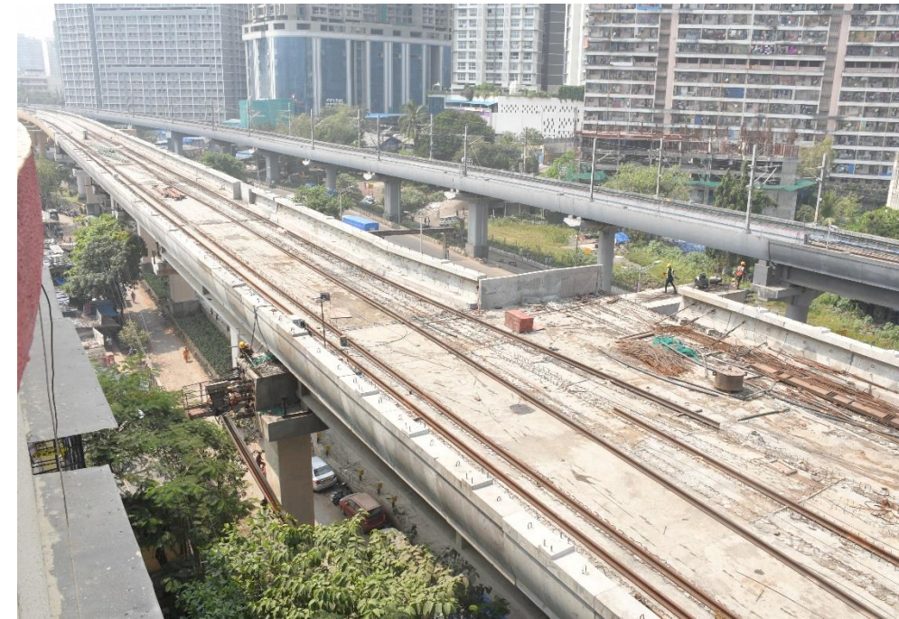
Mumbai Metro Line 9
