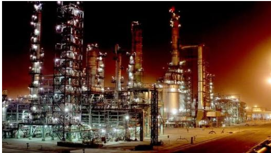
IOCL Gujarat Refinery
