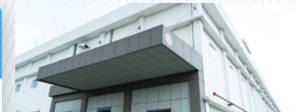
State-of-the-art T20 US FDA accredited solid dosage manufacturing facility at Panoli, Gujarat
