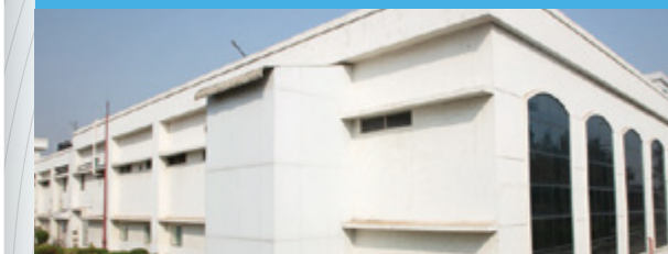
State-of-the-art Ti-10 US FDA accredited solid dosage manufacturing facility at Panoli, Gujarat
